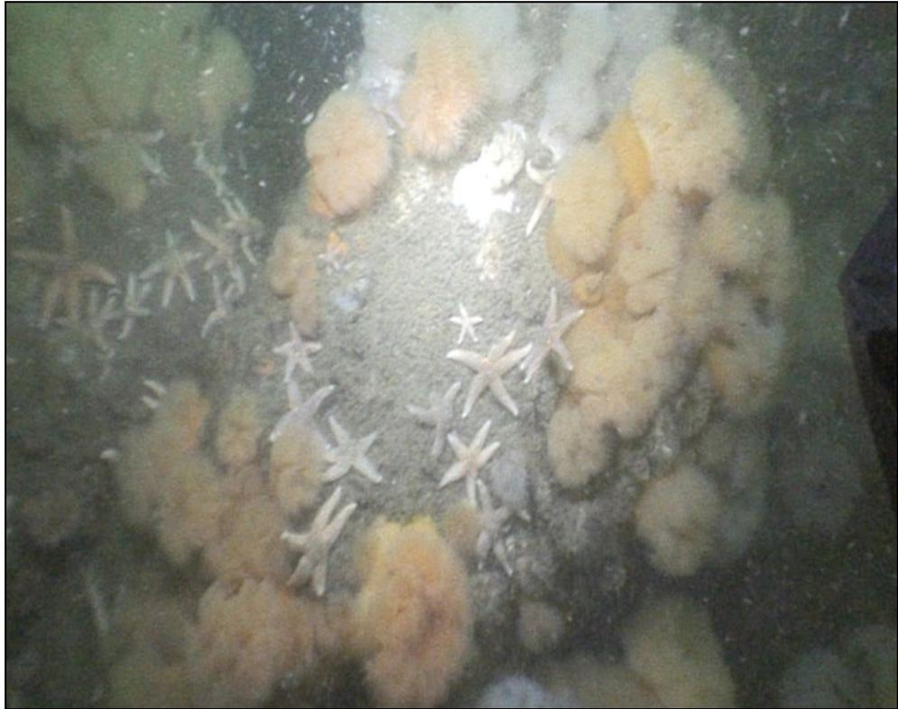
Figure 15. Video still of the scour protection layer of turbine 13 (taken 24<sup>th</sup> of September 2011).
