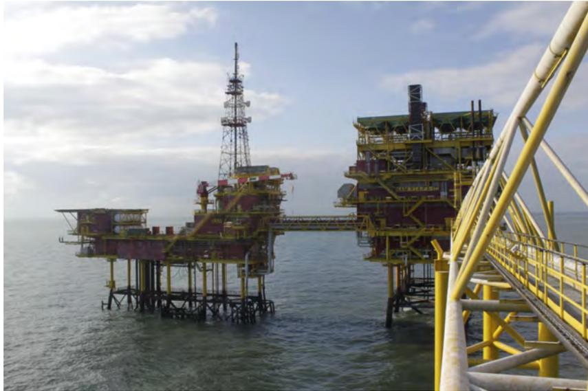
Gas platform K14C of the NAM, as seen looking southwards from the vent stack. Left is the production platform and right the compression platform with the accommodation platform behind it. (photo: Karen Krijgsveld).
